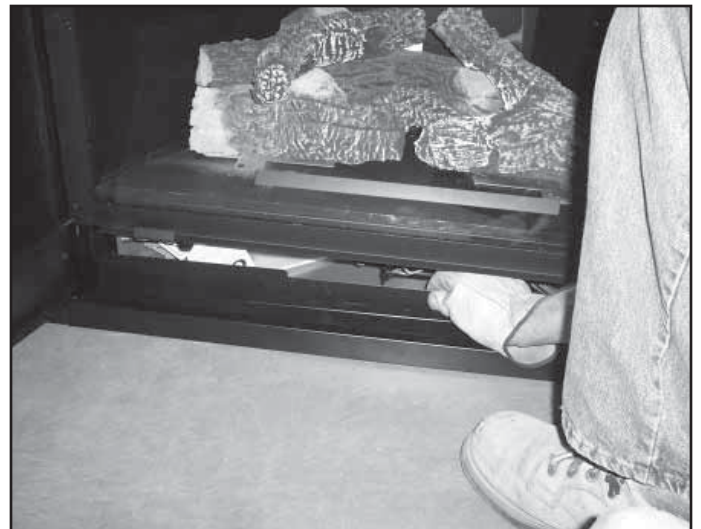
Figure 15.11 Installing Floor Cover
